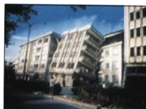
Fig. 2 This inclined building sank unevenly and leans against a neighboring building.
