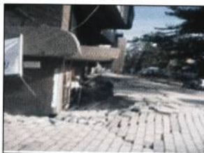
Fig. 1 The Building Sank evenly about 1 m due to soil liquefaction. The displaced soil caused a bulge in the road.
