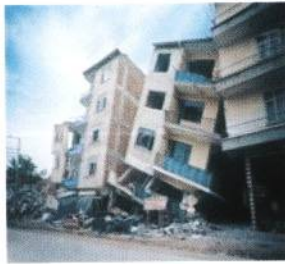
Fig. 4 Sway mechanisms with soft storey ground floors (Izmit, Turkey 1999)
