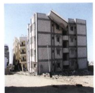
Fig.10 5 storey R.C., collapse of open plinth, water tank at top dislocated)
