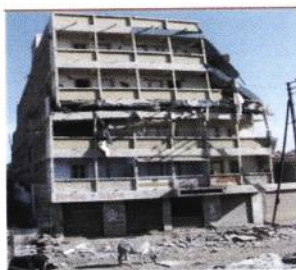
Fig.8:- Collapse of soft middle storey in a building at Bhuj
